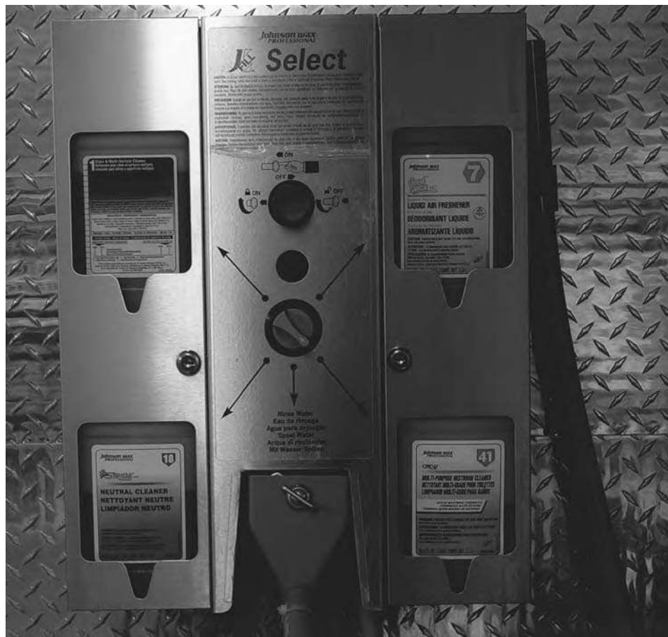
Figure 6-9 A close-up of a chemical mixing station in a satellite linen and storage room. (Courtesy of Bellagio MGM Mirage, Las Vegas, Nevada.)
